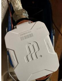
Old water meters are being replaced with new Cell equipped Ultra sonic Badger Meters
