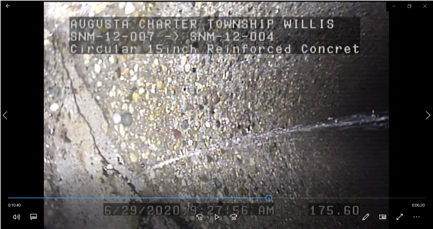
Post-Condition SNG - 1005 Augusta to Meridian, Grouted Runner @ Lateral & 4 Other Locations
